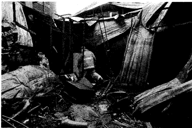
Raleigh Fire Department members walk through the debris of the boiler room assessing the damage. PHOTO BY STEVE WILSON
