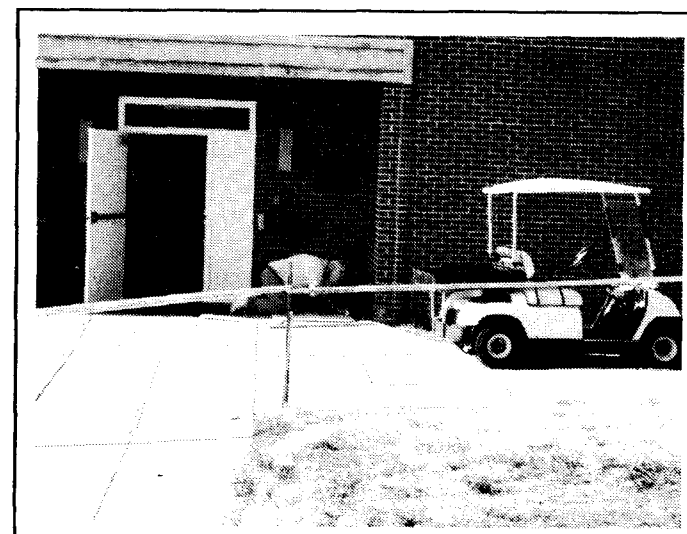
The Barefoot side of Heilman residence hall is closed until more damage can be repaired.
