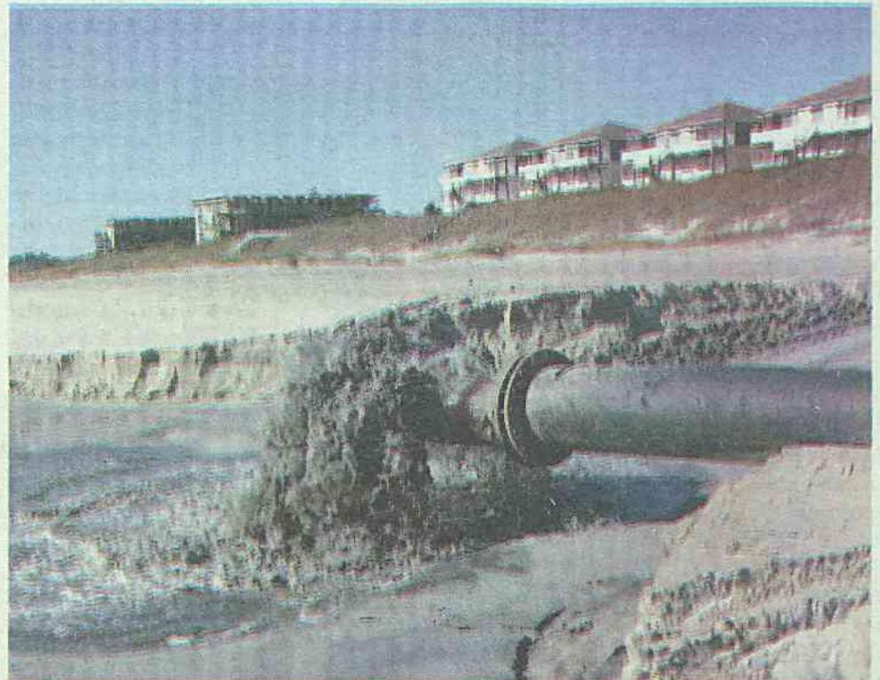
**And It Comes Out Here** – A slurry of sand and water gushes out of the oceanfront end of the pipeline carrying shoal material dredged from sections of the Intracoastal Waterway in Bogue Sound across Bogue Banks for deposit on the ocean beach in Pine Knoll Shores. Some 11,000 truck loads of sand are scheduled to be spread across a 2,000-foot section of beach at the extreme eastern edge of the town.
