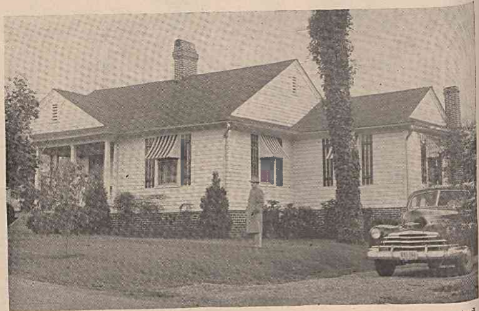
YARD WAS LANDSCAPED , built up two feet and a concrete block wall constructed on upper side. Lower part of lot was leveled off for a graveled driveway. Attractiveness of house exterior was enhanced by gutters and metal awnings and blinds.
