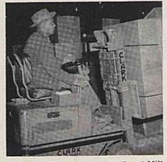
Manuel M. Spencer, of the Towel Mill Shipping Department, operates a battery-powered lift truck to pick up cartons of towels from the conveyor at the end of the packing line and deliver them to the proper storage location in the warehouse. When orders are being shipped, he removes the proper cartons from storage and delivers them to the loading platform as needed.
