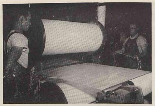
WASTE CONTROL—Preparing to start a new set on a slasher at the Towel Mill, W. O. Haden (right), slasher tender, and John Akers, slasher helper, pull lease strings as close as possible to the point where the set has been tied on. This assures that only a minimum amount of hard waste will be made. The proper start-up of new sets is one of the easiest ways that slasher operators can help reduce losses from waste.
