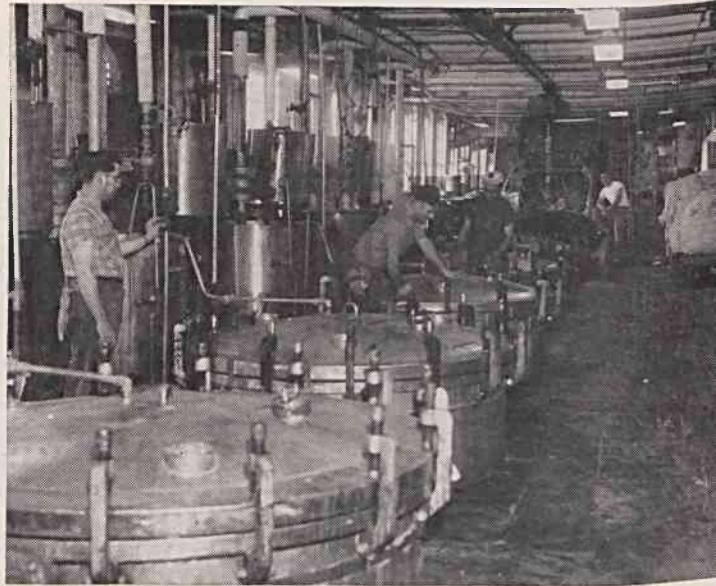
In Dyeing Department, unneeded skein dyeing equipment removed; "drug room" was built for dyes and chemicals.
