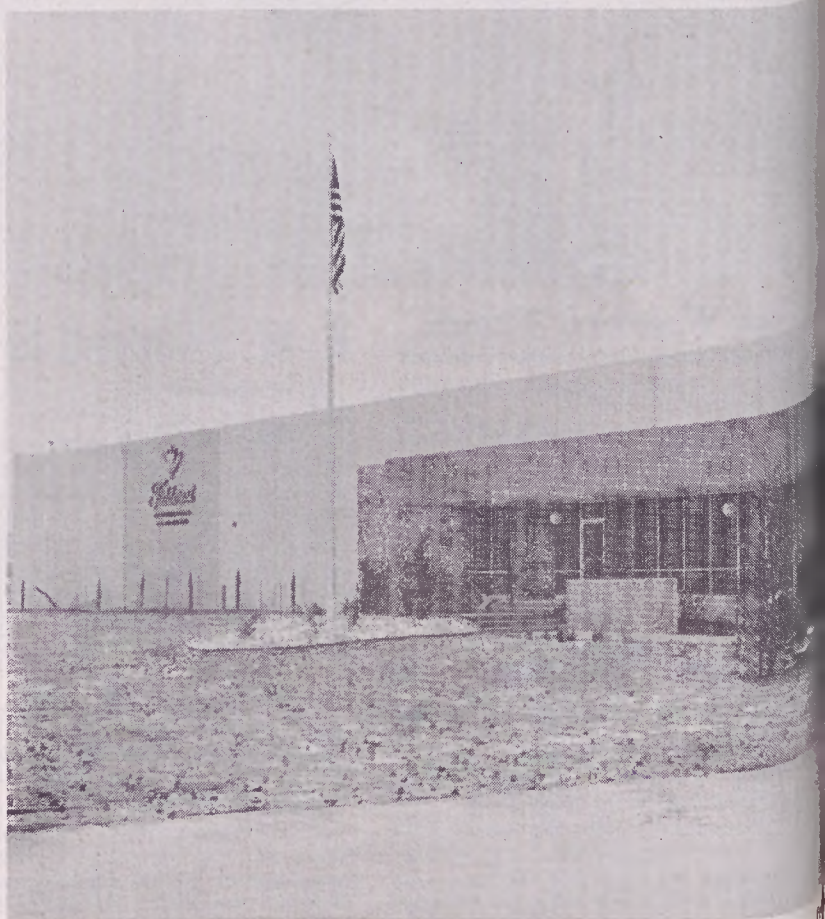
New Fieldcrest Service Center in Los Angeles affords facilities
