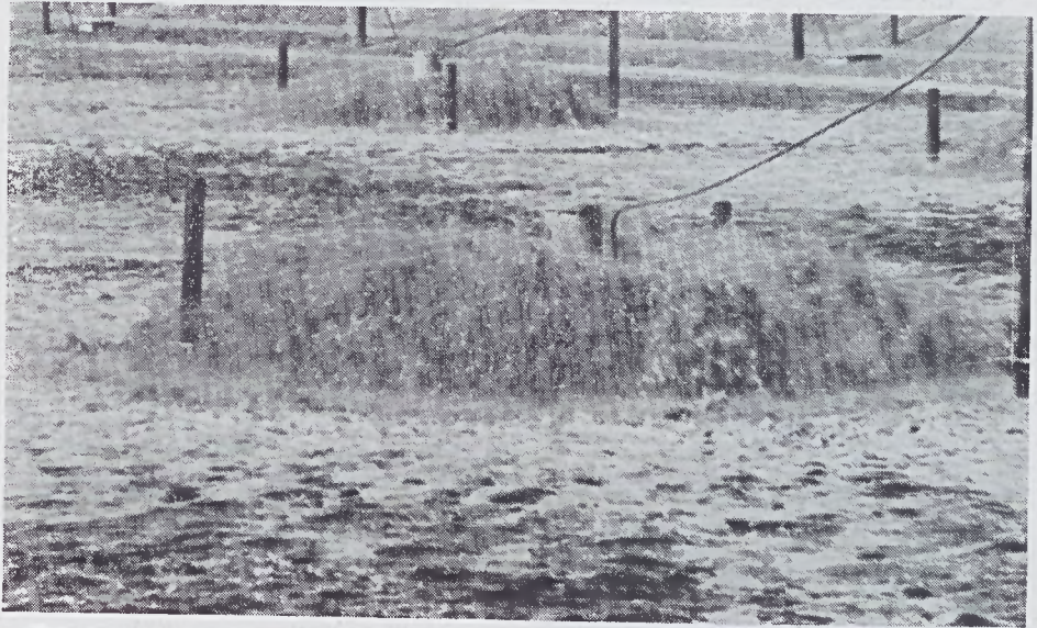
This is close-up showing spraying action of aerators at waste treatment plant.
