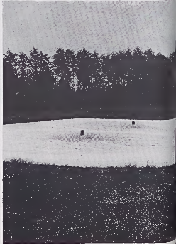
One of the lagoons used for aeration. In this important water treatment process, large aerators throw the sludge into the air enabling it to pick up oxygen.
