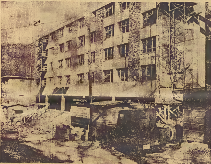
NEW WOMEN'S RESIDENCE HALL
