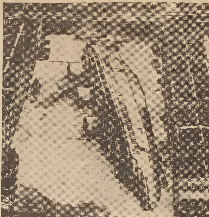
Pictured from the air is the charred, blistered hulk of the former luxury liner, Normandy, more recently the U. S. naval auxiliary Lafayette, as she lay on her side at the North river berth in New York, after capsizing. Weight of the water poured into her holds during a five-hour blaze caused the great ship to turn over.
