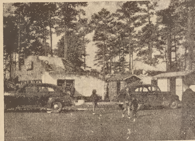
GURKIN'S FILLING STATION —Located south of the tavern. A number of persons in this building at the time of the explosion were injured. The station and cabins nearby were practically destroyed.
