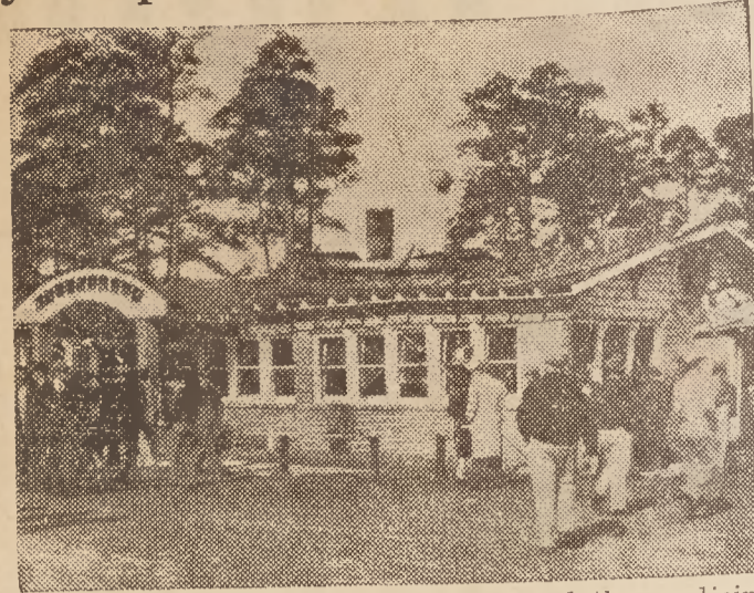
GURKIN'S TAVERN —This building and those adjoining were totally demolished. Several of the employees and a number of guests in the building at the time of the blast were injured.
