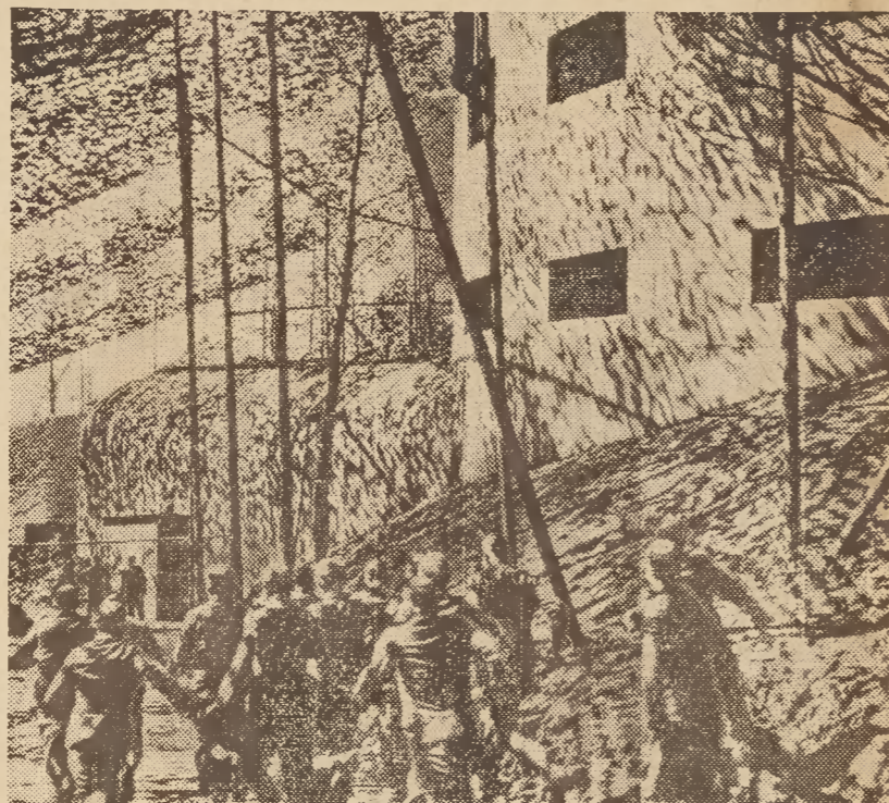
The first picture to be published in America of the concrete and steel "fort" which the occupying Germans have built on the French coast at the point where the English channel is narrowest. The "Toll battery," as it is called, is manned day and night and is camouflaged. Here Germans who man the guns have been given the alarm signal and are dashing for their posts.
