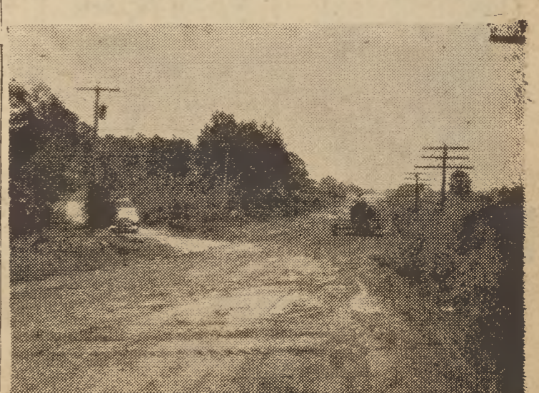
The above photo shows a new road being cut along the Southern Railway in Wilson's Mills. The new highway will connect with the old Loop Road that goes by Miss Bet Vinson's farm and then into the Prison Camp. A car can be seen coming out of the old road to the left. The highway machine to the right is a road scraper.
