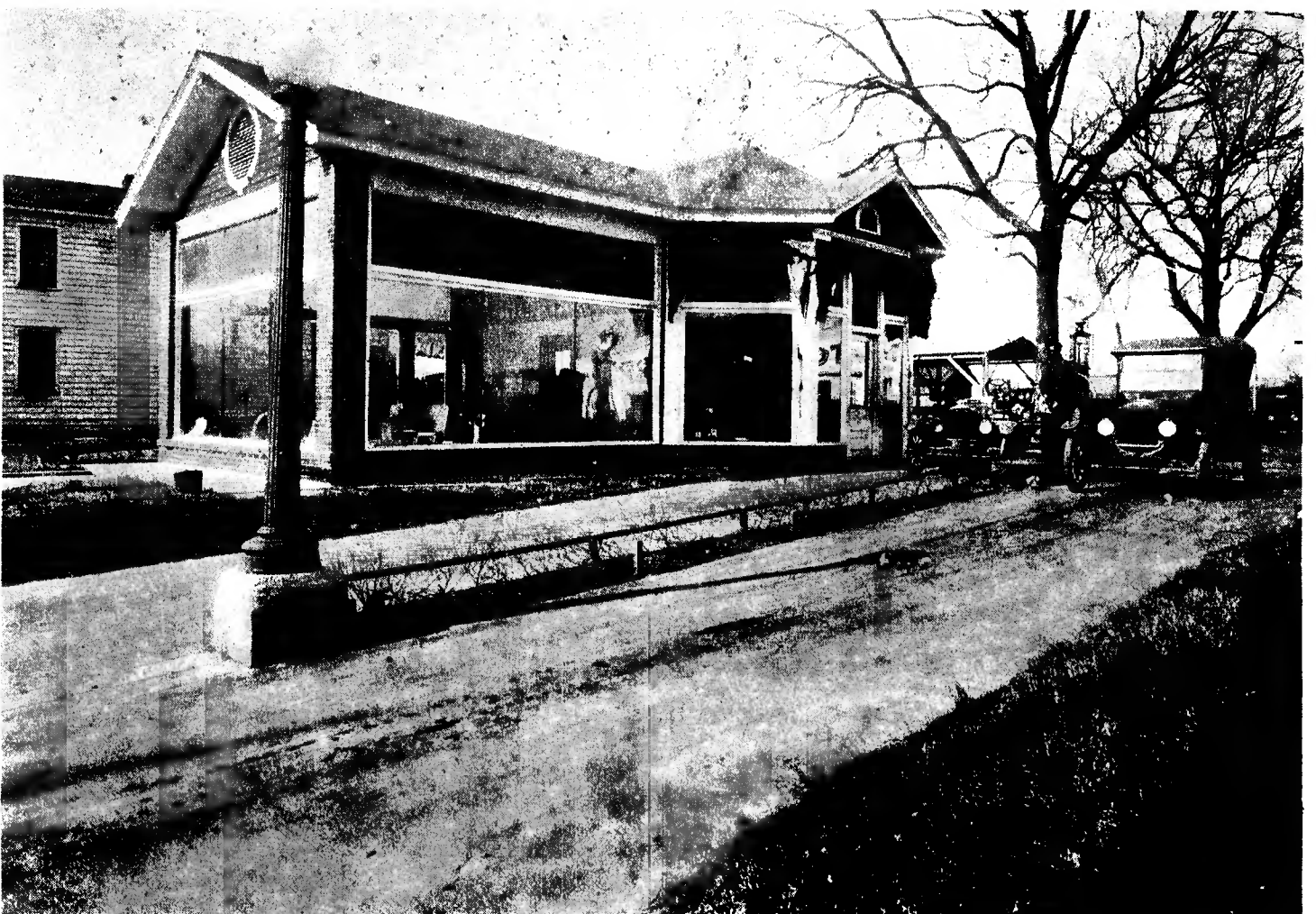
HERE IT IS—Where else but in The Mirror would you expect to find a photograph of the very first drive-in service station built in New Bern? Erected and operated by John H. Parker on what is now the Seashore
