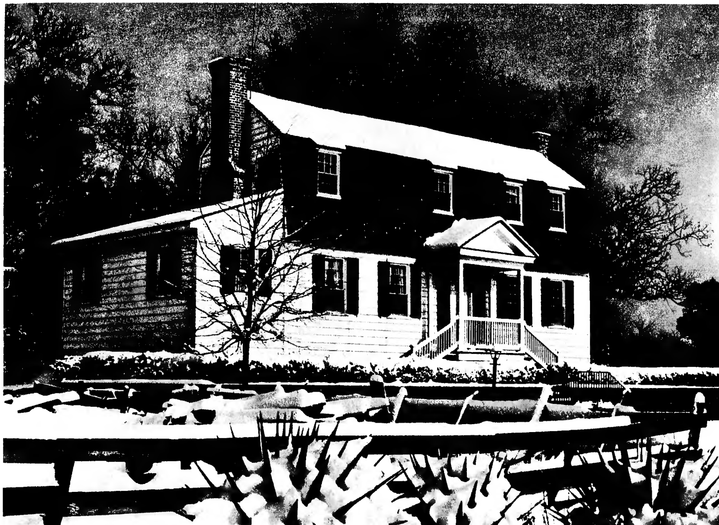
TOPPED WITH FROSTING—Visitors and home towners alike admire the attractive frame dwelling that Ben and Charlotte Hurst live in at Gull Harbor on upper East Front street. Owned by Dr. Charles Ashford, it was moved intact from upper Pollock street
