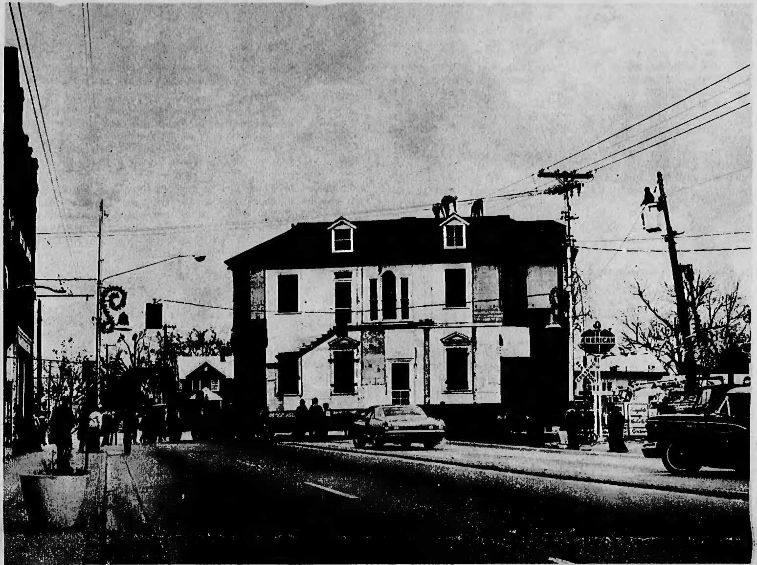
ON ITS WAY—New Bern's historic John Wright Stanley home, where George Washington slept while visiting our town, rounds the intersection of Hancock and Broad Streets, enroute to the new location selected for it on George Street near Tryon Palace. Note work-
