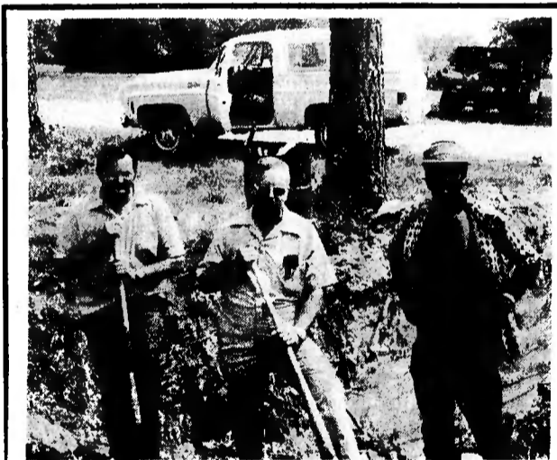
CONSTRUCTION SITE— Vanceboro Mayor Jimmie Morris (center) checks on the construction being done on Hwy 17 from Grand Avenue to the city limits. Crews with the L. A. Reynolds Construction, Co. have been installing drainage pipes in preparation for curbing and guttering.
