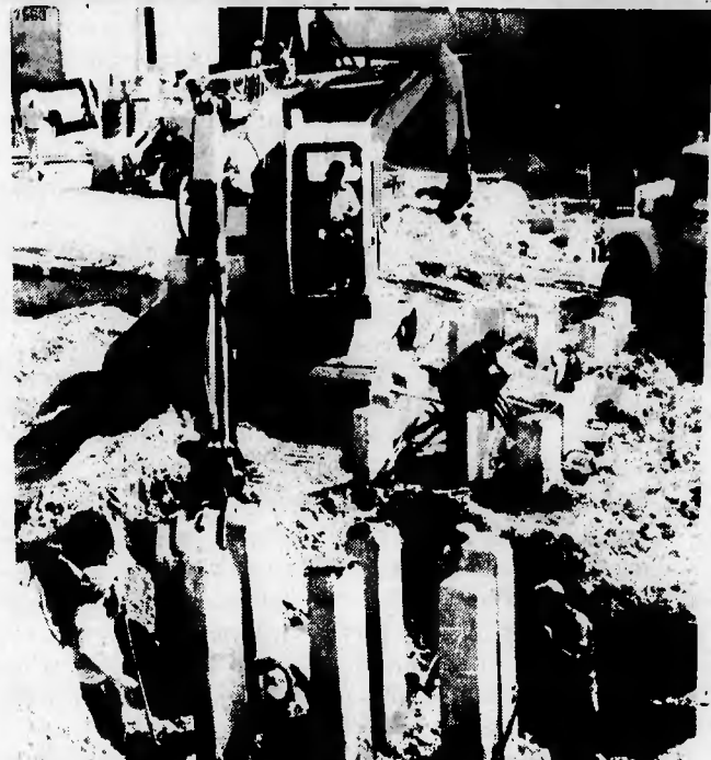
Vanceboro construction crew makes sure the new Craven County Jail is built on solid foundation. Pictured above is Jimmy Morris, Drott operator; in the hole L-R: Terry Morris, Don Lilly, Charlie Ipock.
