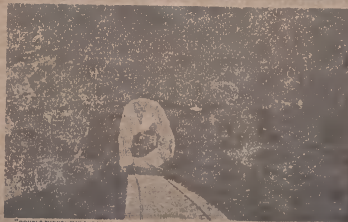
Climbing the Blue Ridge, the train passes through seven tunnels, of which the Swannanoa is the longest. This tunnel extends 1,823 feet under the Assembly grounds, at a depth of 123 feet.
