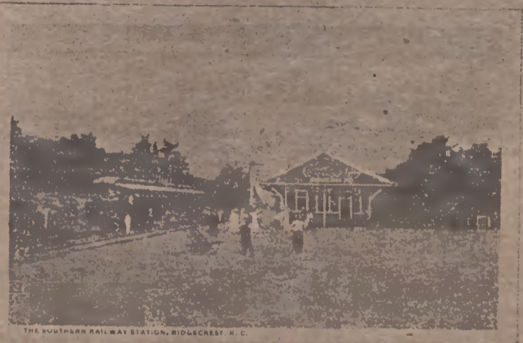
The Railway Station at Ridgecrest, on the top of the Blue Ridge Mountains, is a short distance west of the Swannanoa Tunnel. Eight passenger trains stop here daily. One mile west is Mt. Mitchell Station, from which passenger trains make the ascent to Mt. Mitchell, the highest mountain east of the Mississippi River.
