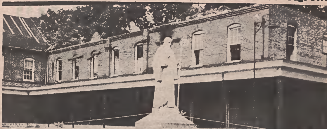
St. Benedict stands before the roofless, boarded up Brother's Building, which burned during Easter Week 1960.
