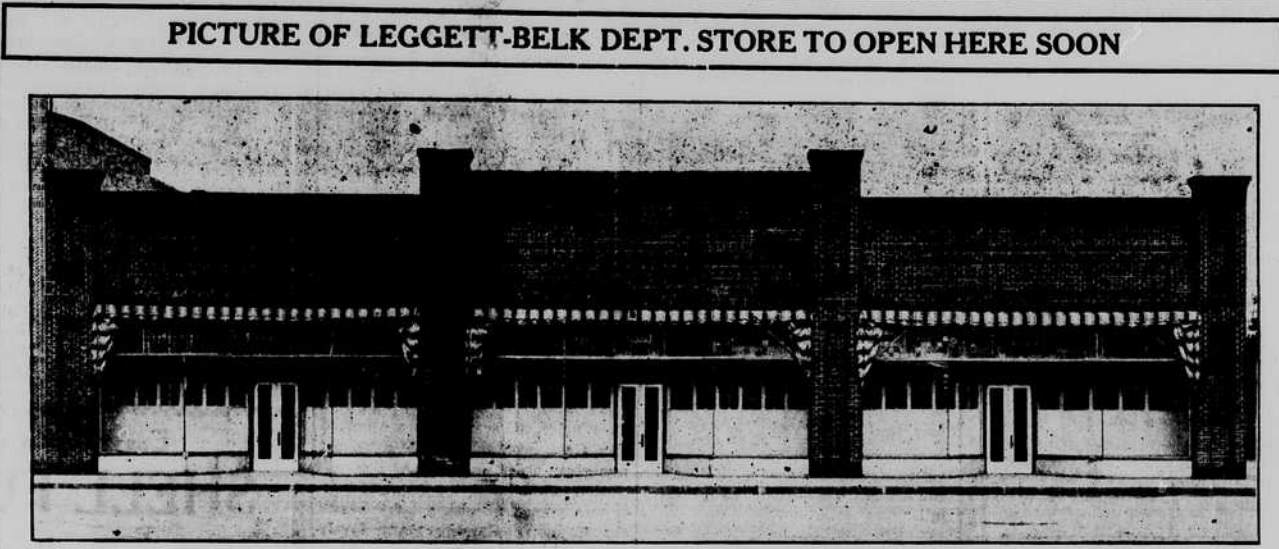
This will be the home of the Leggett's Department Store, which will open here for business in the near future. The huge building is being remodeled thruout. The new fixtures will be installed next week. The location is at the corner of Roanoke Avenue and 11th Street.
