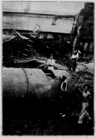
Scene at J. R. Wollett Lumber Co. in Littleton, taken shortly after the terrific boiler explosion recently which cost one life and did damage to the mill plant estimated at \$25,000. Mark Jenkins died the same afternoon from burns received when scalded by steam. He was dragged from the debris and rushed to the hospital.
