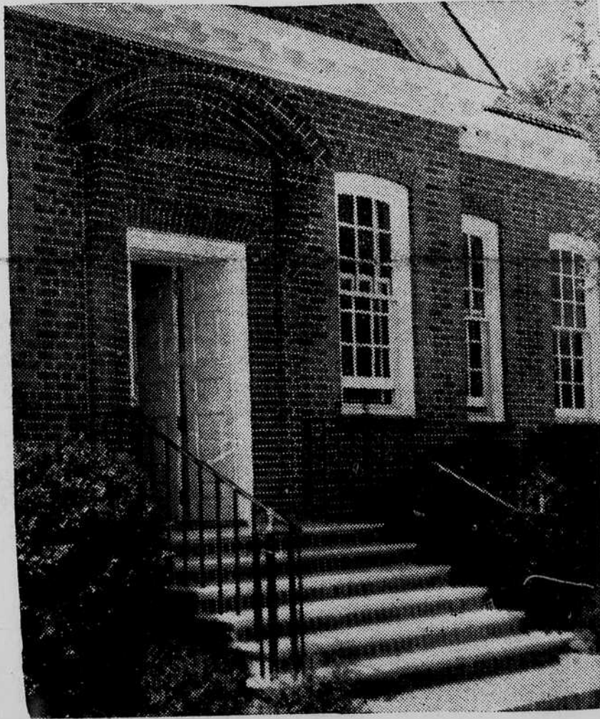
Above is a close-up of the door opening on Fifth Street in the recently completed office building for the Roanoke Mills Company here. Photo shows the brick work, iron railing, marble topped steps, door panelling—all colonial Williamsburg designs.
