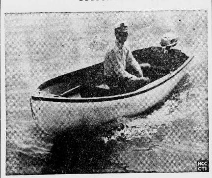
When scientists put cotton and plastics together the result is a cotton boat. Made from plastic laminated cotton, this boat, complete with all fittings, weighs less than 150 pounds, the National Cotton Council states. Since the hull of the boat is molded in one piece, it is watertight. Easily handled by two persons, the cotton boat will carry up to six 200-pound adults or eight youngsters.
