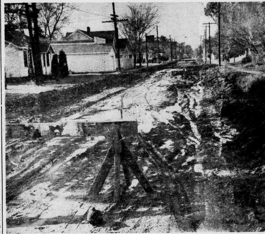
This picture taken one block east of the 10th and Hamilton Street crossing, shows the new 10th Street extension in a muddy condition after the rains last week. Now undergoing preliminary grading, prior to paving, the extension, when completed, will provide a shorter route to and from the Weldon-Roanoke Rapids highway and will tend to speed up traffic at the Junction. (Present plans of the board of city commissioners call for a traffic light to be placed at the 10th and Hamilton crossing, shown in the background).
