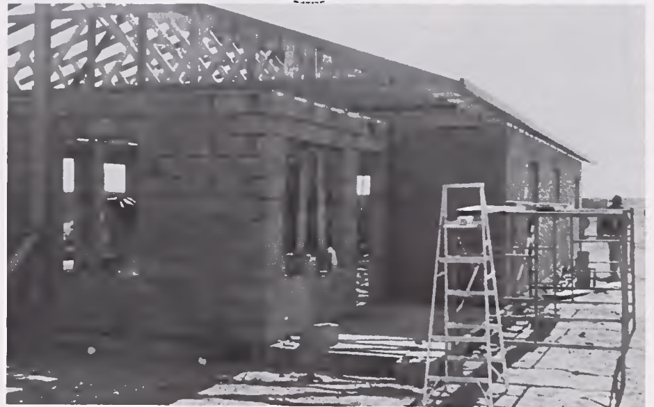
One of two buildings nears completion.
