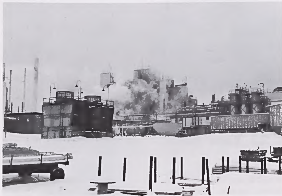
Clouds of vapor almost obscure CP on this cold day. At present, there's no practical way to recover this low grade lost heat.
