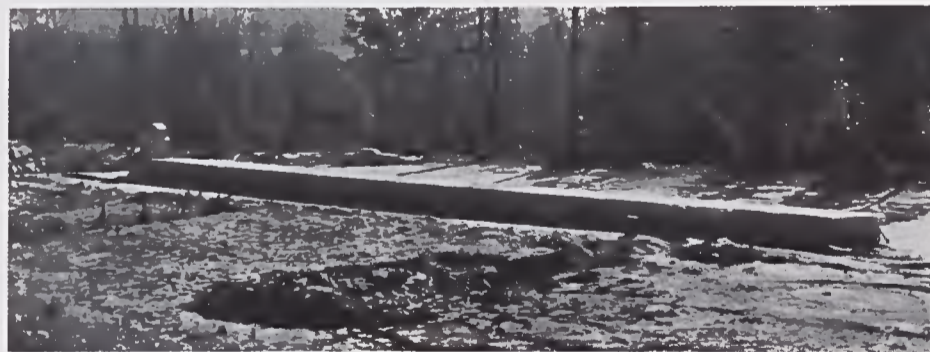
Solar Sludge Dryer
