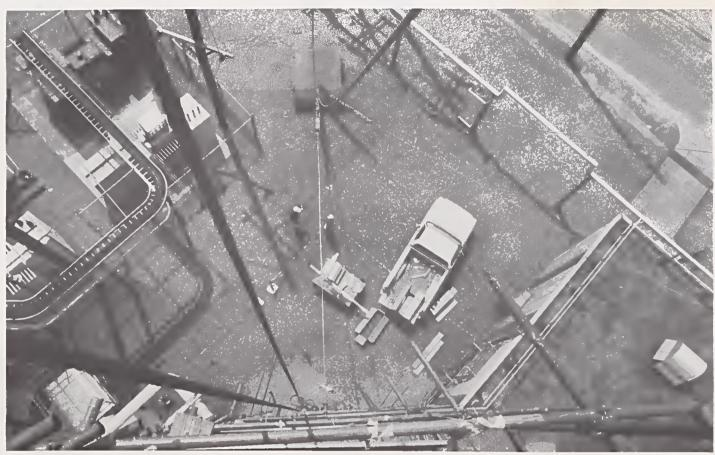
**REACHING FURTHER** for energy savings takes on new meaning from the viewpoint of the man up the stack at the powerhouse. Insulating the stacks is part of the work required to install economizers on the steam boilers. This project will save an estimated 250,000 gallons of fuel per year, according to the project engineer, Jack Harron.
