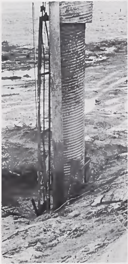
A BROKEN VALVE drained DERA Lake and launched a two day effort to save the fish.
