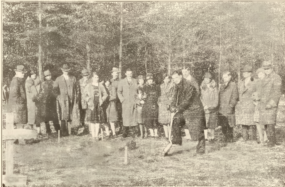
Student representatives and officials present at the ground breaking were, reading from left to right: E. D. Broadhurst, chairman of the board of education; Mrs. C. T. Lipscomb; not identified; C. L. Jacobs, representing Angle-Blackford Construction Company; not identified; Rachael Lipscomb, girls' athletic representative; Annette Donavan, president semester 8; not identified; Bill Petree, boys' athletics; Melisse Mullens, student; Miss Fannie Starr Mitchell, dean of girls; Elizabeth Boyst, Girls' Council; Louis Brooks, Homespun ; Miss Mary Morrow, president of Faculty Club; Carl Jones, president of semester 7; H. S. McCray, associated architects; Clyde Norcom, High Life ; C. W. Phillips, acting superintendent of city schools; and in the foreground, Charles Rives, president of Student Council, digging first shovel of dirt.
