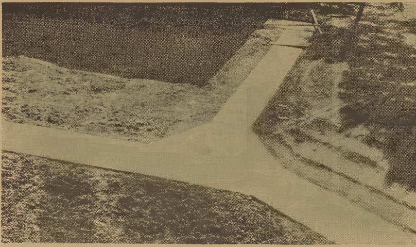
"The above picture is of the new walkway built by the Junior Civitan Club. The concrete takes the place of the infamous 'Okeefenokee Swamp.'
