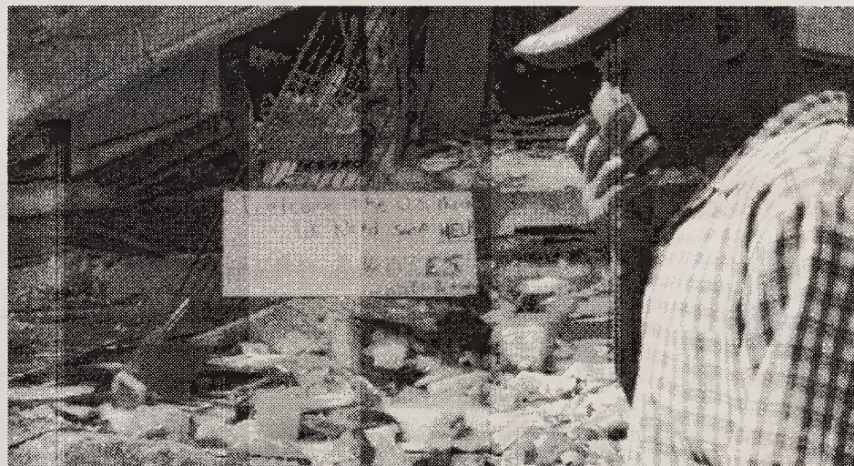
A Haitian walks past a collapsed building after the 7.0 M earthquake struck the capital Port-au-Prince. A sign reads, "Welcome the U.S. Military. We Need Some Help. Dead bodies inside." Internet graphic
