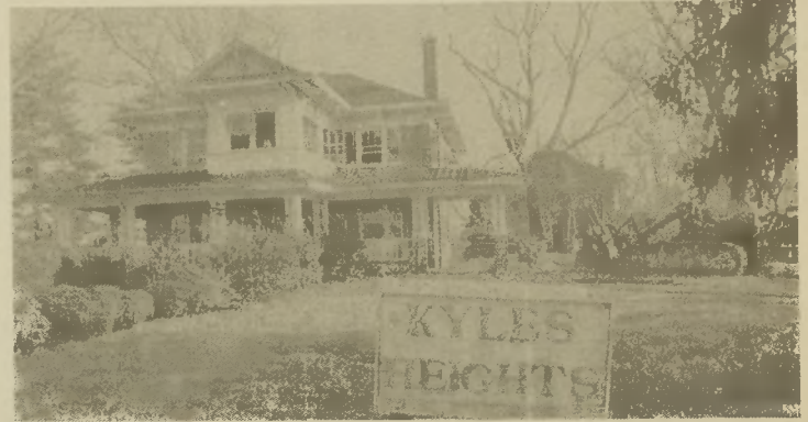
Kyle Heights was a failed attempt at low-cost housing for senior citizens. It was leveled on March 25, and Charlotte diocese has no immediate plans for the property.
