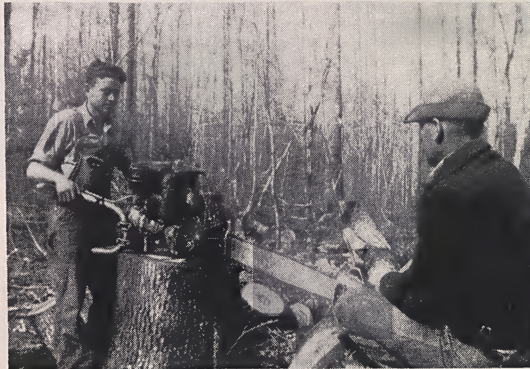
Willie Clifton Joyner (Weaveshed) operates a chain power saw during his spare time. In this picture he is assisted by his son, Boice, and Willie Williams. Clifton said he can cut five cords of wood per hour. He charges $4.00 an hour, and it is a right profitable business except when a chain breaks and he has to buy a new one for $25.75.
