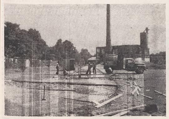
Two new gateways have been installed giving access for entrance and exit on West Elm Street. These gateways are joined by a 14' x 741' long concrete roadway. The area around the frame repair building and the rear of the boiler plant will also be covered with concrete. One of the main purposes of this new construction is to provide easier access to the frame repair building and boiler plant area. It also connects with our present shipping road and can be used in conjunction with this.
