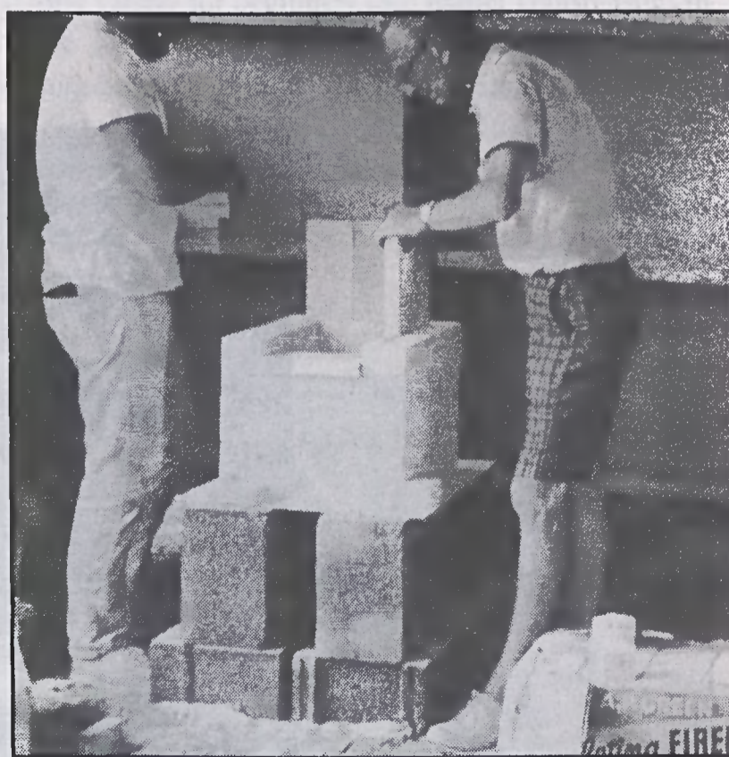
Construction of the annealer in the first glass studio in 1965
