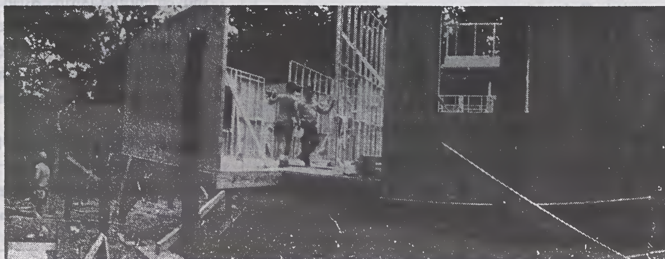
Construction of ADA housing
