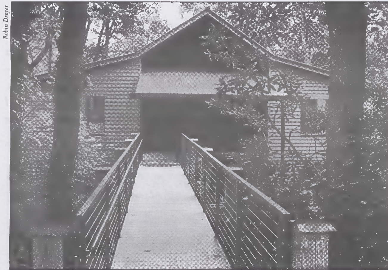
Dorm 54, designed by architect Dail Dixon, was built with funds raised as part of the Preserve Penland campaign. The steel caps on the posts were designed and made by resident artist Marc Maiorana.
