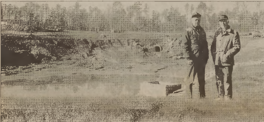
THE DOWNSIDE OF DEVELOPMENT—Bill Buchanan and Bill Clark, left and right, are unhappy with erosion they contend will only get worse as Perimeter Park is developed above their properties.
