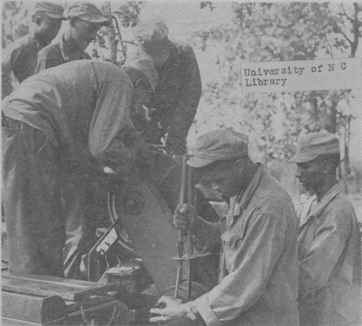
Members of the Fortieth Signal Construction Battalion took part in the Army's giganite maneuver, "Southern Pine," which is now underway in the sandhills area of
