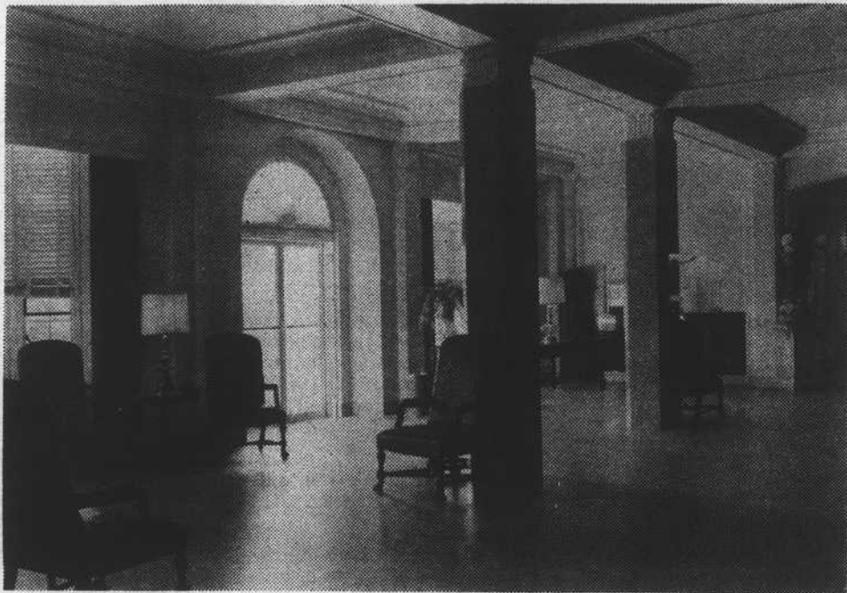
IN NEW LOBBY — Shown is the main entrance lobby at St. Joseph's Hospital, just inside the new south entrance, with new terrazzo floor and marble paneling. The whole first floor has been completely renovated. (Story and photographs through the courtesy of The Sandhill Citizen, Aberdeen, N.C.)
