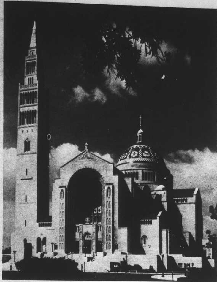
EXTERIOR VIEW of the National Shrine of the Immaculate Conception, at Washington, D.C., which is developing a patina now that it has been exposed to the elements for some years, bringing out in greater detail some of the elaborate carving and statuary with which it is adorned. (NC Photos)
