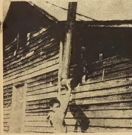
Defective Flue Damages House
