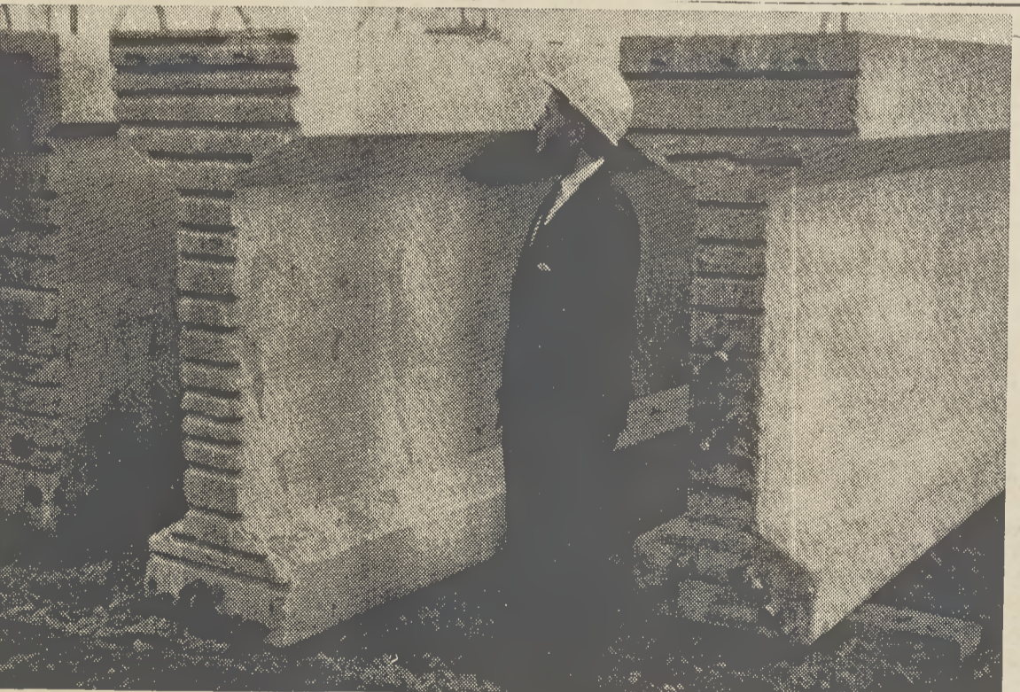
Athey Vice-President, Assistant to the President, Paul Linney is shown inspecting concrete post tension roof beams that weigh 70 tons last January. There are five such beams, each made up of five sections, placed 51 feet high to form an assembly and welding section of the sprawling Wake Forest Athey plant. —(Photo by Bob Allen).
