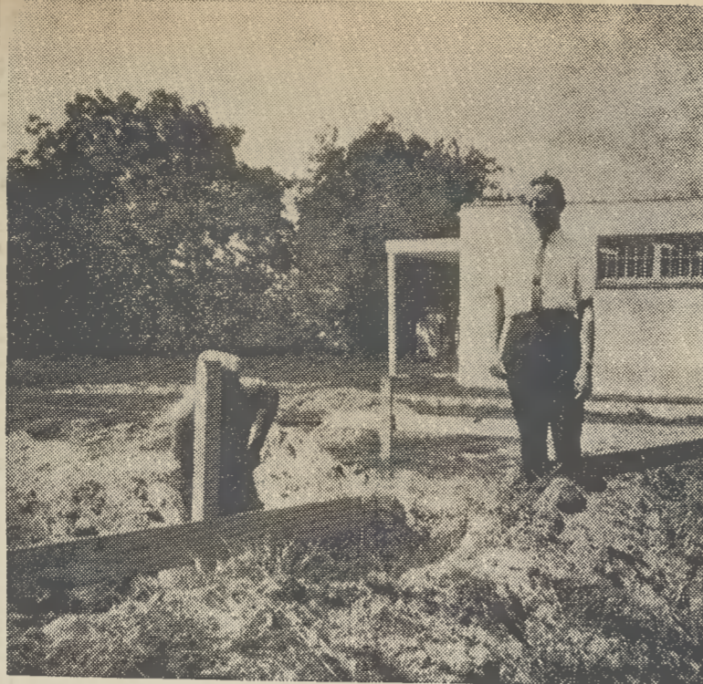
Curtis Underwood looks over construction — (Lois Barham Photo).
