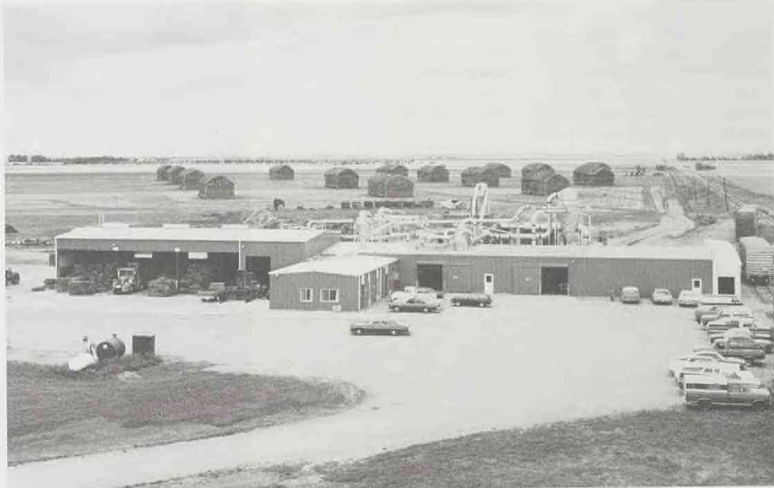
The decortication plant is located in Watertown, South Dakota. At this plant, the woody portion of the flax stalk is removed in preparation for shipment to Pisgah Forest where cigarette and specialty papers are made. Note the bales of flax in the background. In the off season, the plant-fibre operation employs approximately 200 people while as many as 600, during the months of April through November, are employed.
