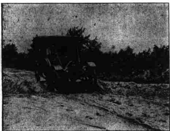
Fig. 2. Road with steep grade (average 10 per cent.) Travel made more difficult by uneven surface of road; large stones project above the road.
