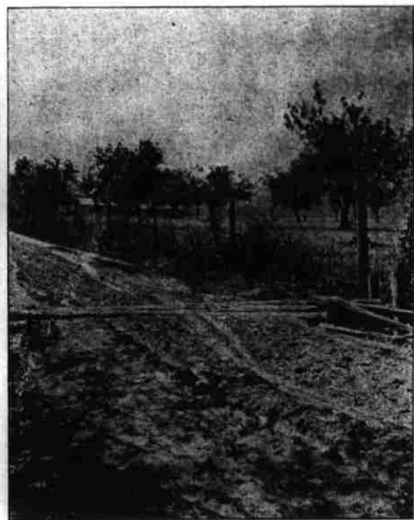
Fig. 4. A Craven County Culvert, Old Style, Regular Vehicle Smasher.
